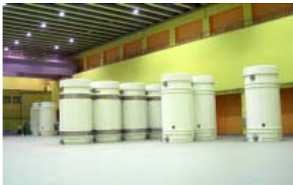
Centralised dry store for casks of HLW, the Zwiilag facility, Würenlingen, Switzerland
